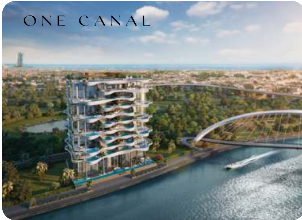
DUBAI WATER CANAL
